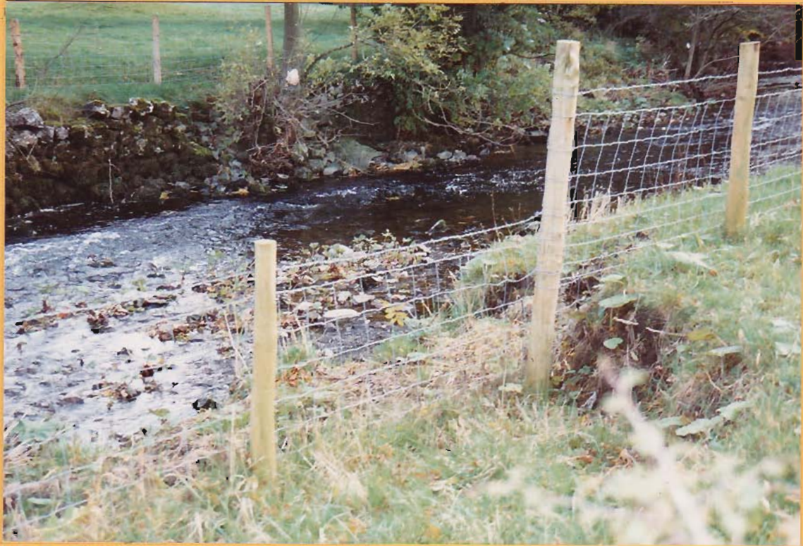
3. FENCE CONSTRUCTION - SHOWING STEPPED FENCE.
