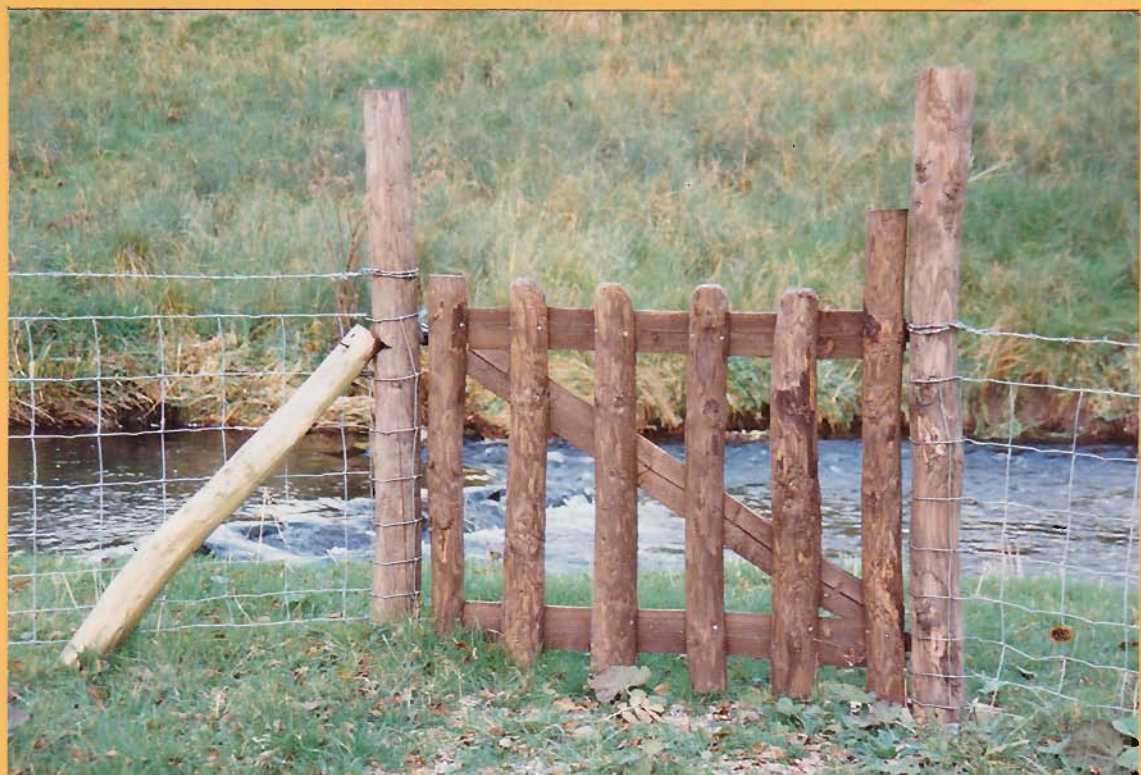
2. GATE CONSTRUCTION - EASTGATE.
